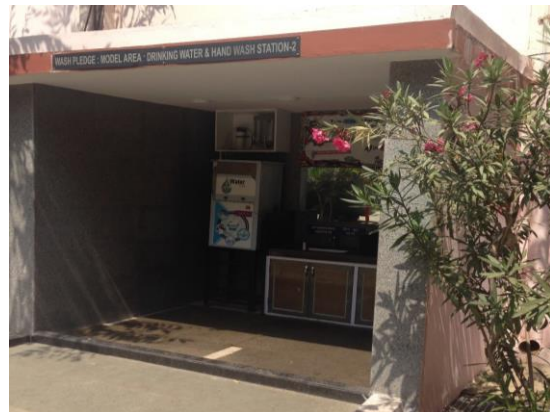
Renovated Drinking Water and Hand Wash Station for Contractor Workmen in their Work Area
